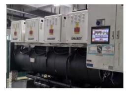
Air pressure system energy saving. The old screw air compressor was replaced with a 10KV high-pressure centrifugal air compressor, efficiency was increased by more than 20%, the system's annual power saving was 2.28 million kWh, and annual carbon reduction was 1,324 tonnes of  $\rm CO_2$  equivalent.
