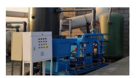
Tunnel oven uses heat pump for energy saving. The oven electric heater was replaced with a condenser, using a heat pump for heating and heat exchange, achieving an annual power saving of 310,000 kWh, and a carbon reduction of 178 tonnes of CO<sub>2</sub> equivalent.
